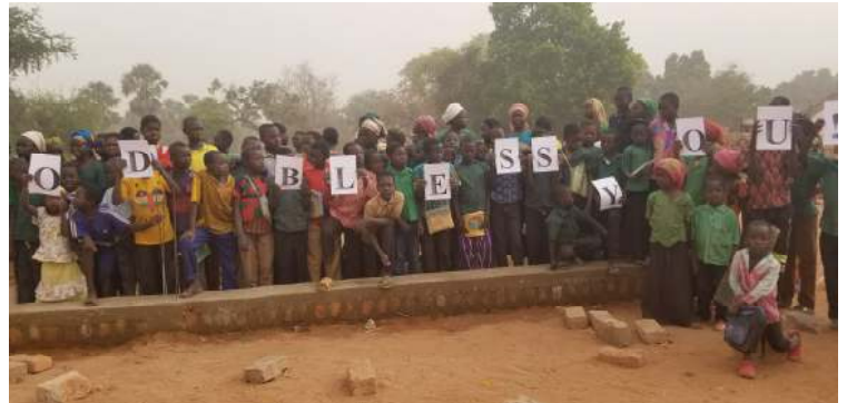
Primary school students standing on the new building foundation, holding sign that reads, God Bless you
